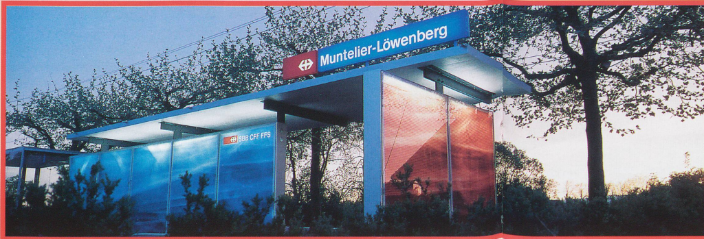
The station - seen here from the street side - lights up in the evening twilight. Photo SBB.
