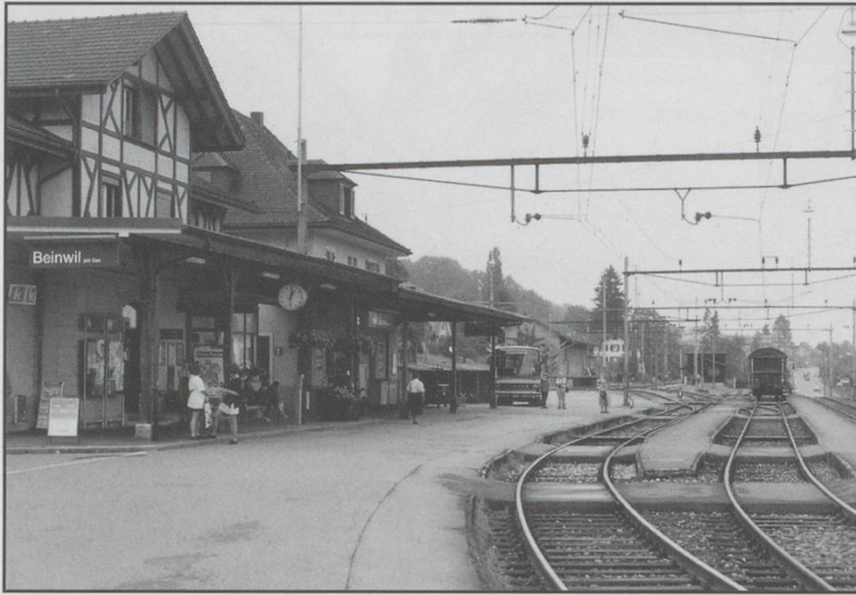
Beinwil in August 1997. LH line was the branch platform. Wagons from the branch are stored in the centre road. Nowadays the RH loop is a truncated siding and wagons are left there, and the further centre road is the main line. A PTT Setra 315 awaits Beromünster passengers from the connecting train. All photos in the article are by Ernie Brack.
