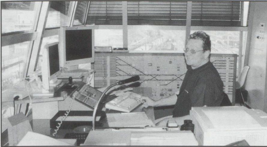
Muttenz, Feb. 2003. Wagon control in the East Signal Tower.
