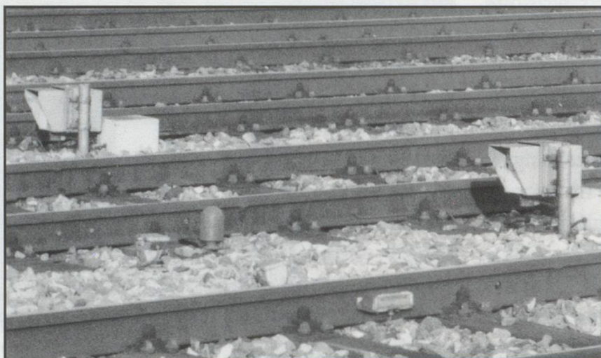
Muttenz. Feb. 2003. Wagon speed detectors, 1 per track.
