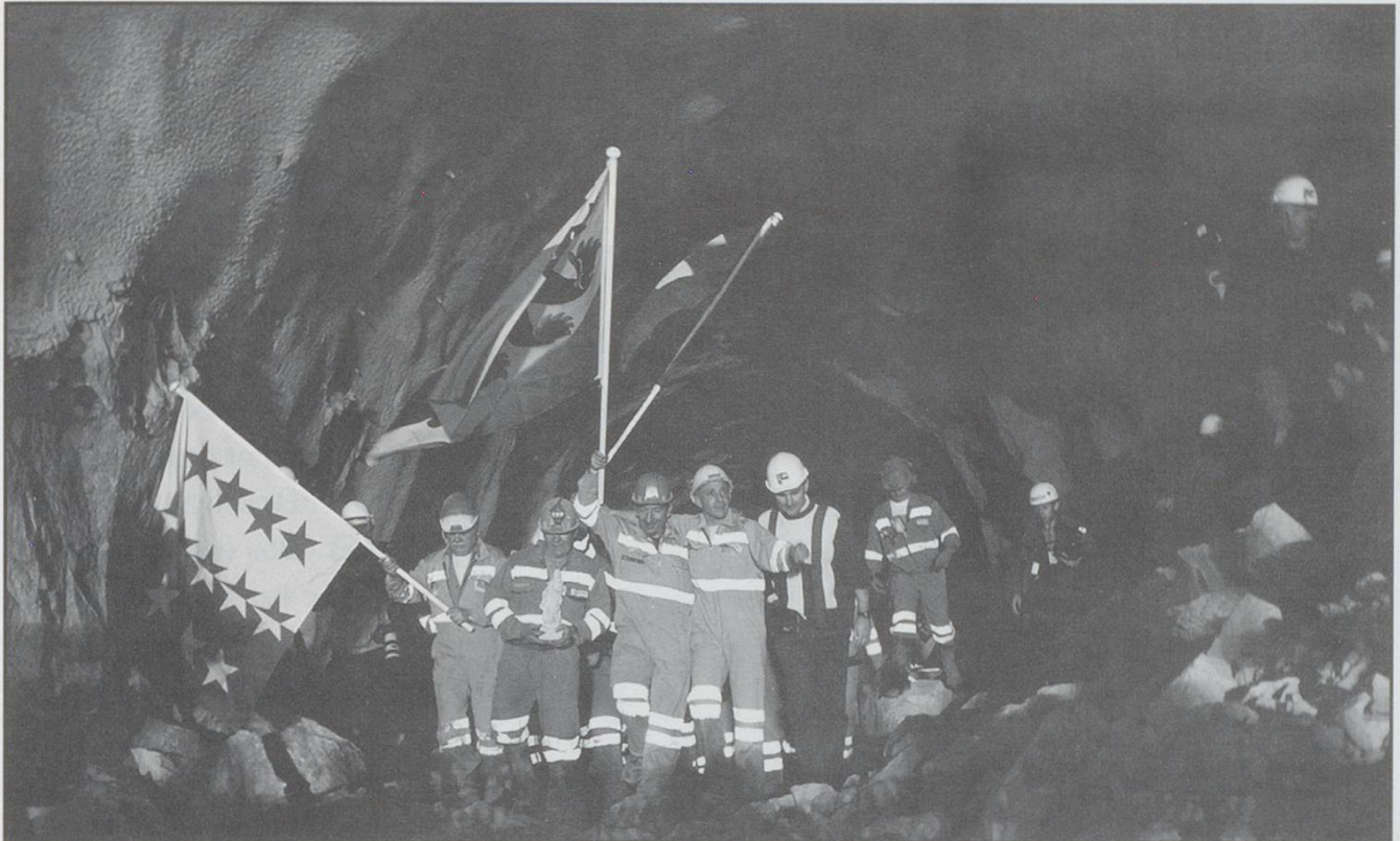
The team from the northern end of the tunnel move forward to meet the teams from the southern end.
