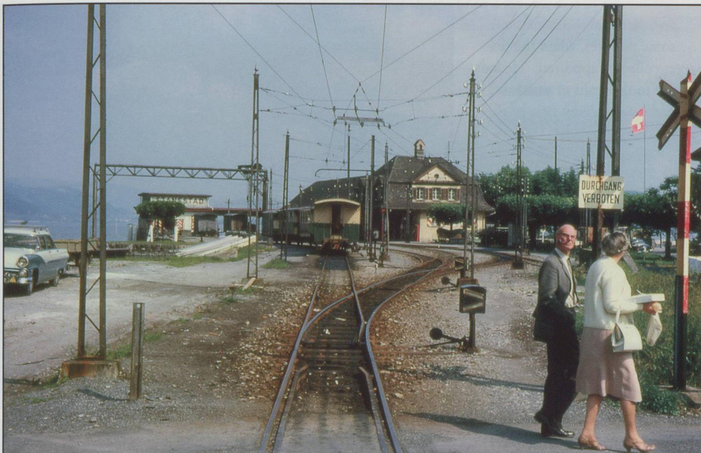
ABOVE: The old line crossing the road into the Harbour Station and the complication of the 3-phase wiring. NEXT PAGE, UPPER: Loco waiting to giving rack assistance. CENTRE: New bridge partially built looking towards the tunnel in 1964. LOWER: Timber false work for the high-level bridge under construction in 1963.
