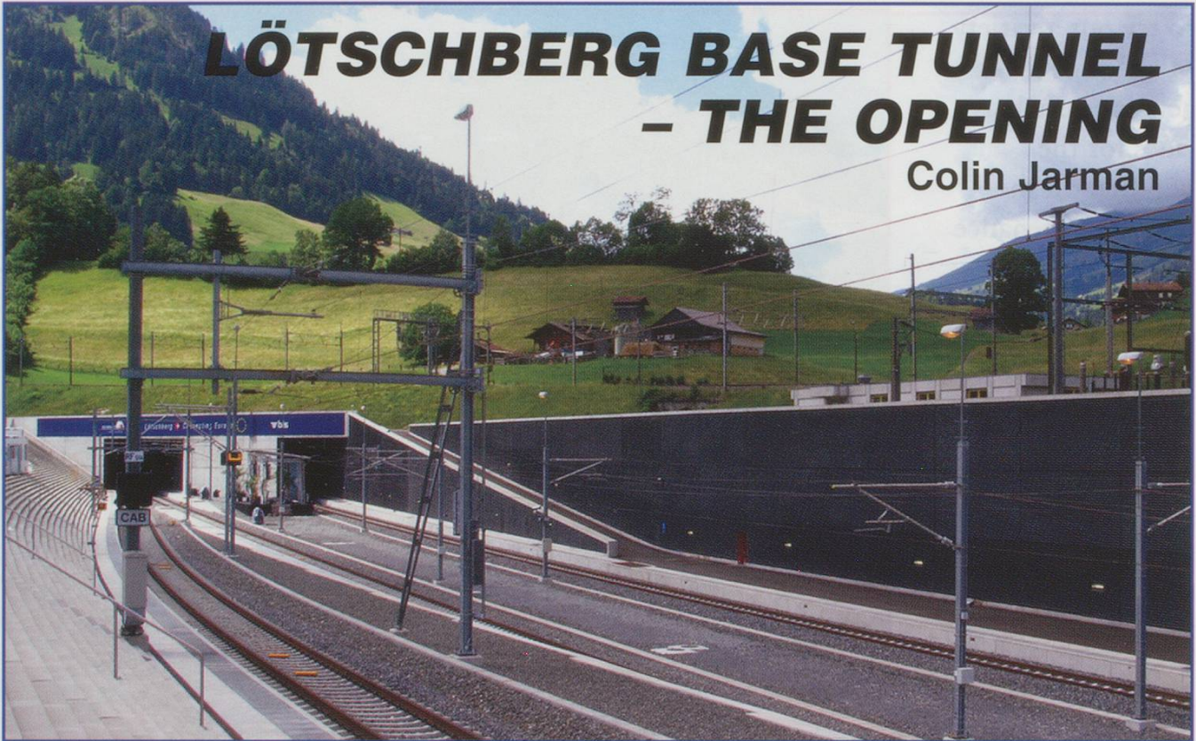
Approach to the Base Tunnel, with a view of the 'mountain route' above. PHOTOS: Colin Jarman
