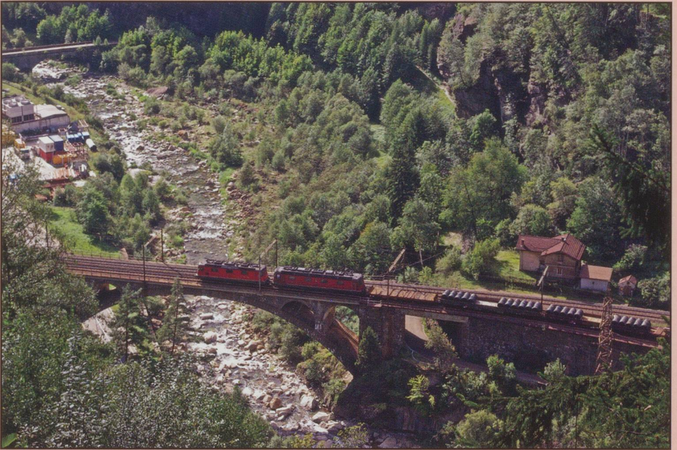
The Polmengo bridge, at the end of the Dazio Grande gorge, can now be viewed from one of the new platforms built for the purpose. As the line runs exactly east/west over the bridge, the best light is early morning in mid-summer.
