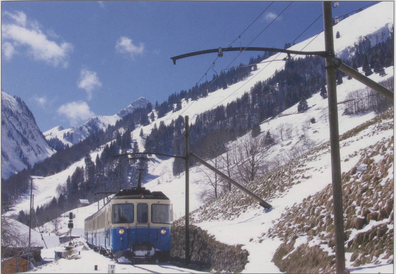
A few remaining wooden overhead poles.
