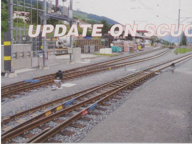
The re-configured yard and turntable at Scuol-Tarasp.
