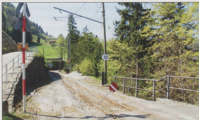
Works on the ASD below La Planches. PHOTO. Jim Cook
