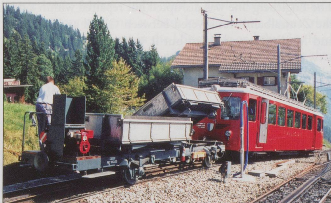
BELOW: Rigi No. 5 tipping building material at Kaltbad.
