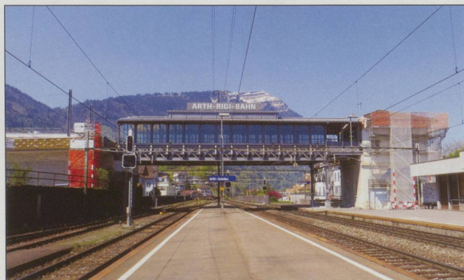
The Rigi station over the main line at Arth Goldau.
