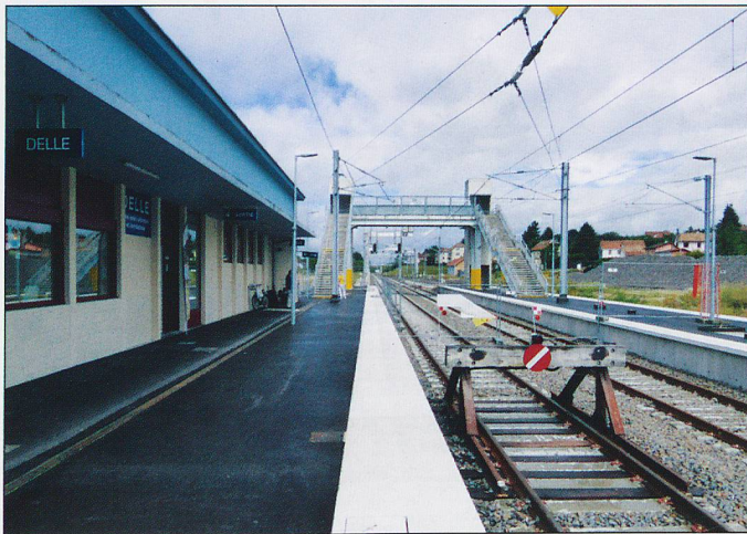
Delle station on the French border on 25 July 2017 with the new extended works for the through services to Belfort, due to start in December this year, clearly seen past the temporary buffer stops. (See 'Swiss News')
