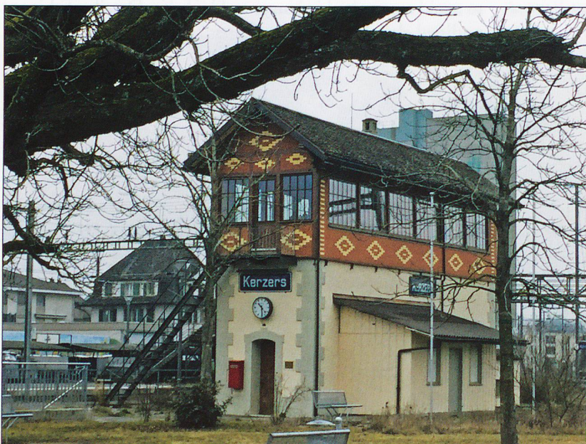
The signal box at Kerzers.
