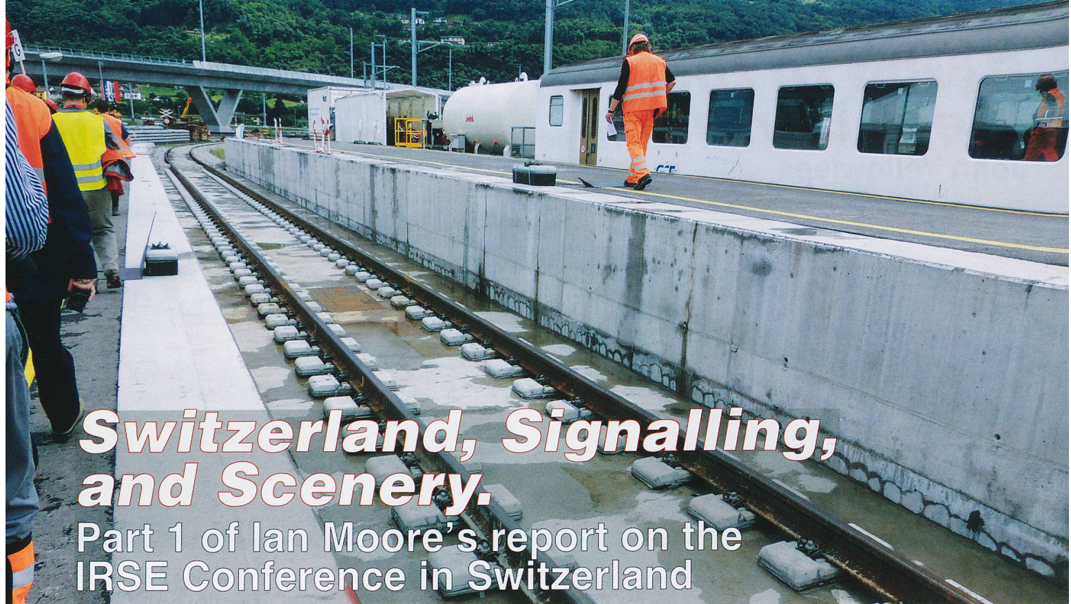
Ceneri Base Tunnel (CBT) north end construction site. A demonstration length of slab track.
