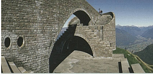
Chiesa di Santa Maria degli Angeli, Monte Tamaro, Ticino. The mountain chapel on Alpe Foppa (1500 m/4921 ft) was built in 1992–96 by Swiss architect Mario Botta.
