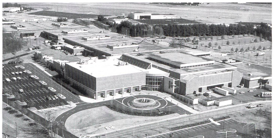
PalmettoExpo Center, Greenville, South Carolina, USA
