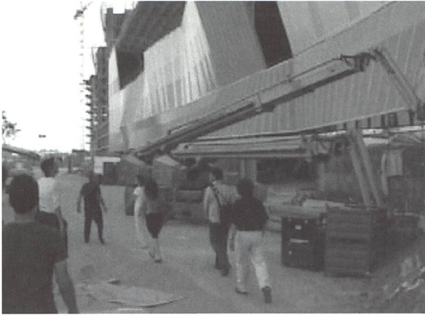
Visit of ETH students to CCIB construction site.
