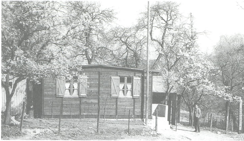
fig. d «Demountable buildings for war victims. 1944/45. [...] Two 6 x 6 m buildings in a Lorraine village.», in: Peter Sulzer, Jean Prouvé, Oeuvre complète, Volume 3: 1944–1954 , Basel, Boston, Berlin 2005, p. 47
