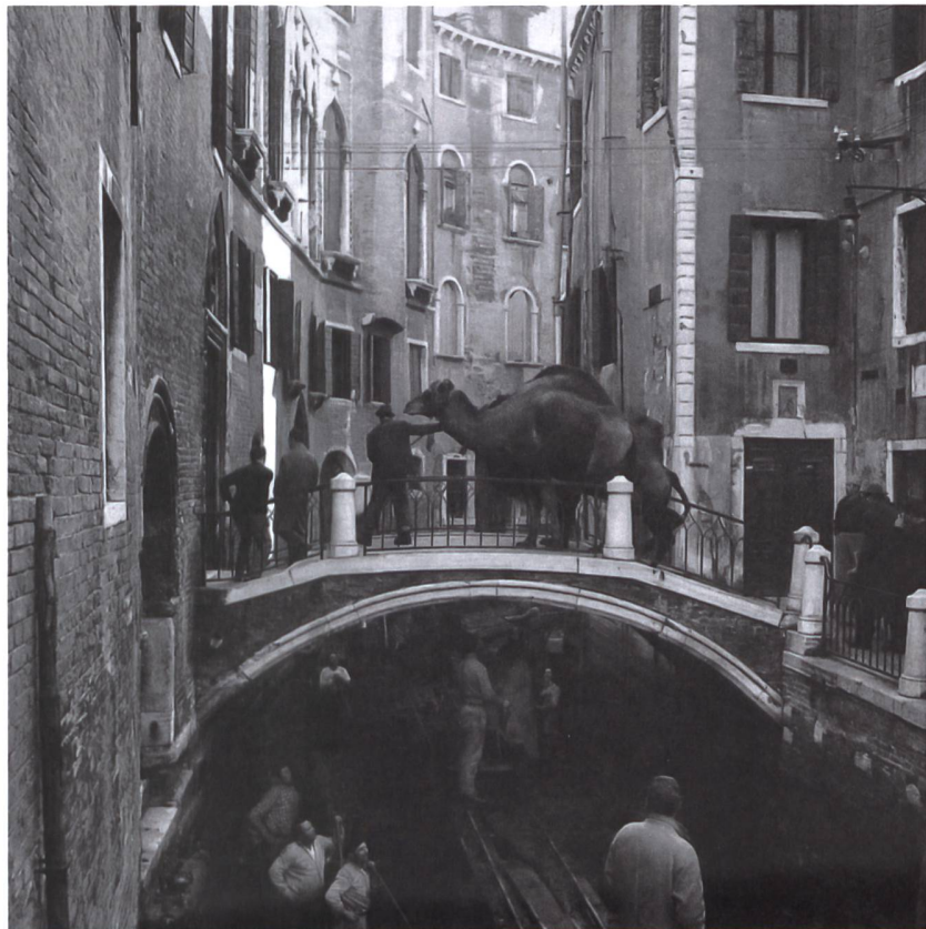
(fig. b) A canal in Venice being drained and cleaned using a Decauville railway and two camels, 1956. Image: Wikimedia Commons
