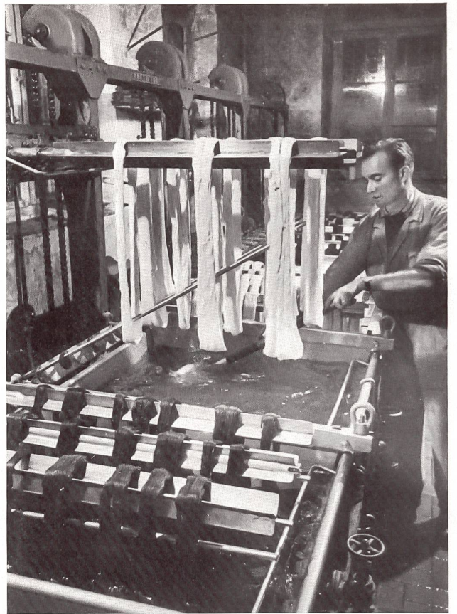
Hank dyeing machine for silk twists.
