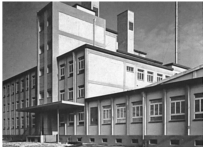
Outside view of the new factory Photo Raoul Heeb
