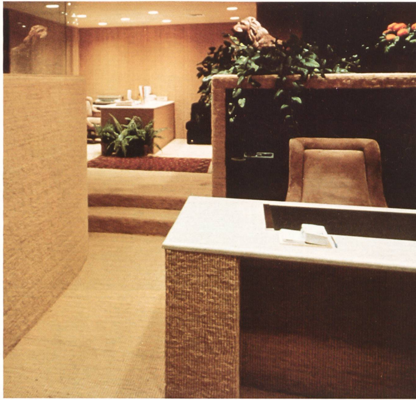
Flame-proof treated sisal matting covers floors and vertical surfaces of desks as well as walls.
