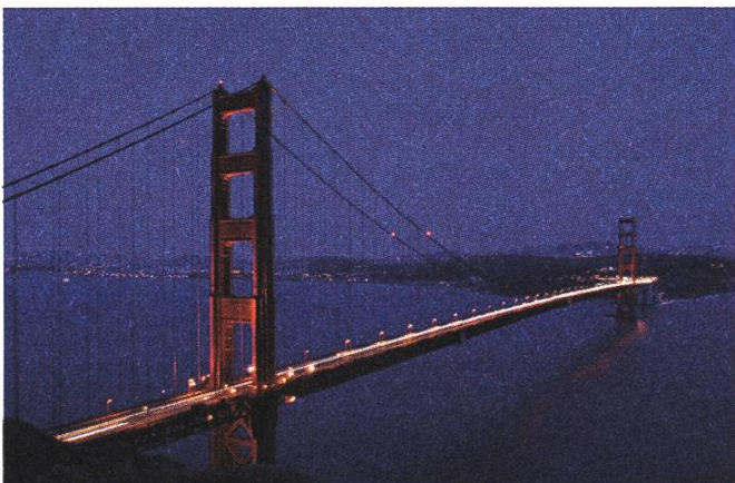
Golden Gate Bridge by night
