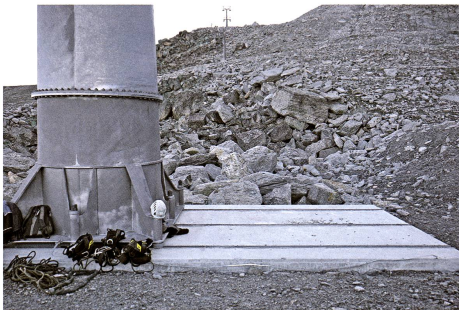
Fig. 9: Chairlift pylon on rails on ice-rich permafrost in a ski resort, Canton Valais.
