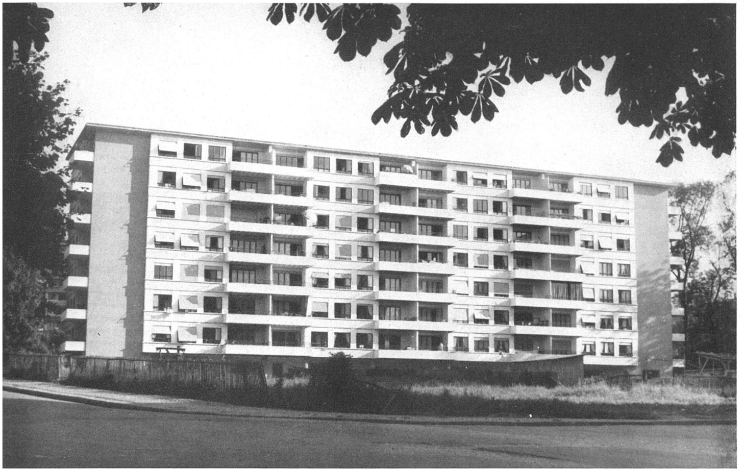
Groupe K 1947/48, façade sud-est / Wohnblock K, Südost-Ansicht / Block of flats K, South-east elevation
