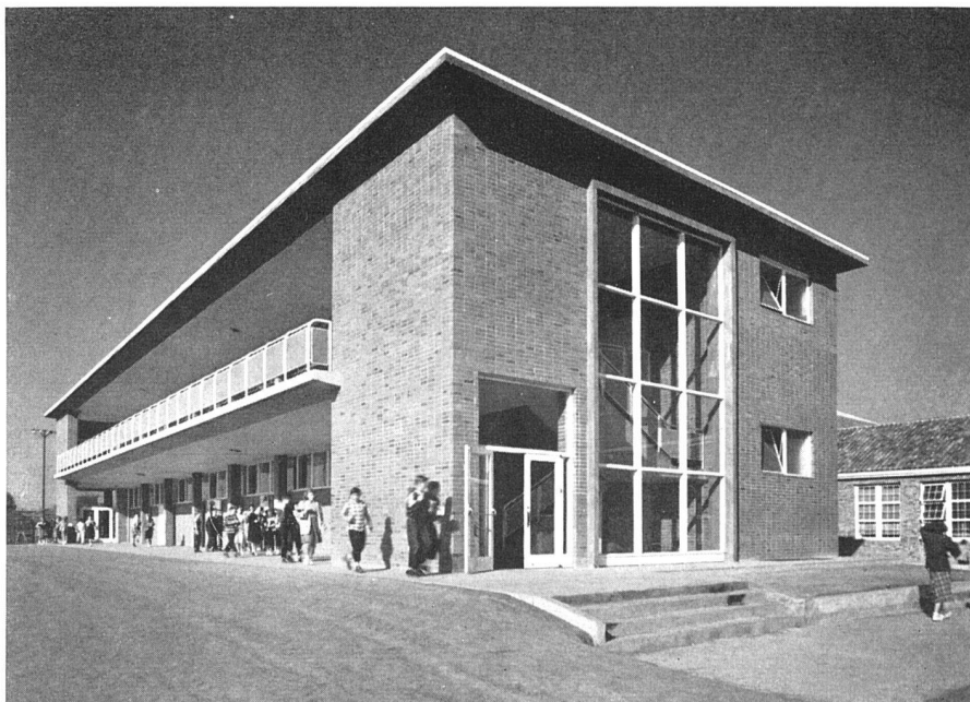
Südost-Ansicht | L'école vue du sud-est | The school from south-east
