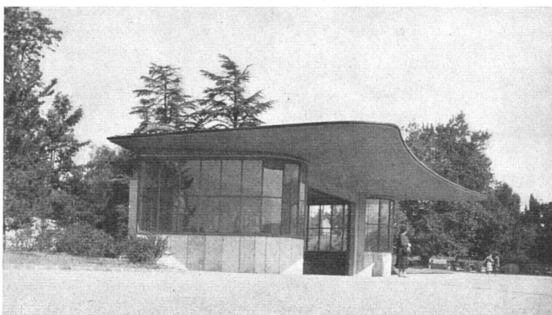
Wartehalle Place des Nations, Genf. 1949, Francis Quétant, Arch. BSA, P. Honegger, Ing. E. I. L., Genf
