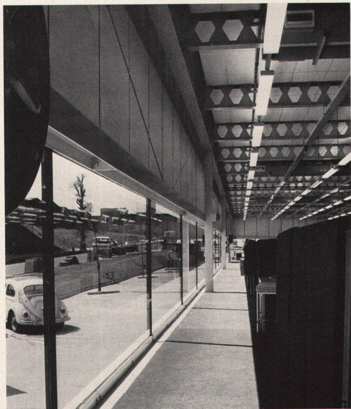
The architects have applied for the research and office building of Computer Technology Ltd in Hemel Hempstead a flexible steel construction system, similar to that presented in the previous publication (332–334). Plywood panels, faced with aluminium on both sides, constitute the upper part of the facades. Neoprene sections serve to insulate the joints
