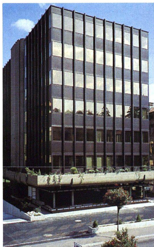
Palazzo Benzug, CH-Lugano, 1977 INFRASTOP-Gold 40/26 Arch. L. Doninelli, Bellinzona
