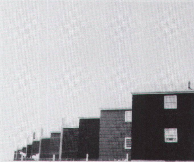
Housing Development, rear view, Bayonne, New Jersey
