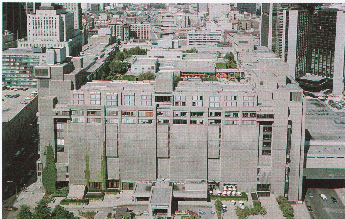
Place Bonaventure; Affleck, Desbarats, Dimakopoulos, Lebensold et Sise, architectes associés, 1964–1967
