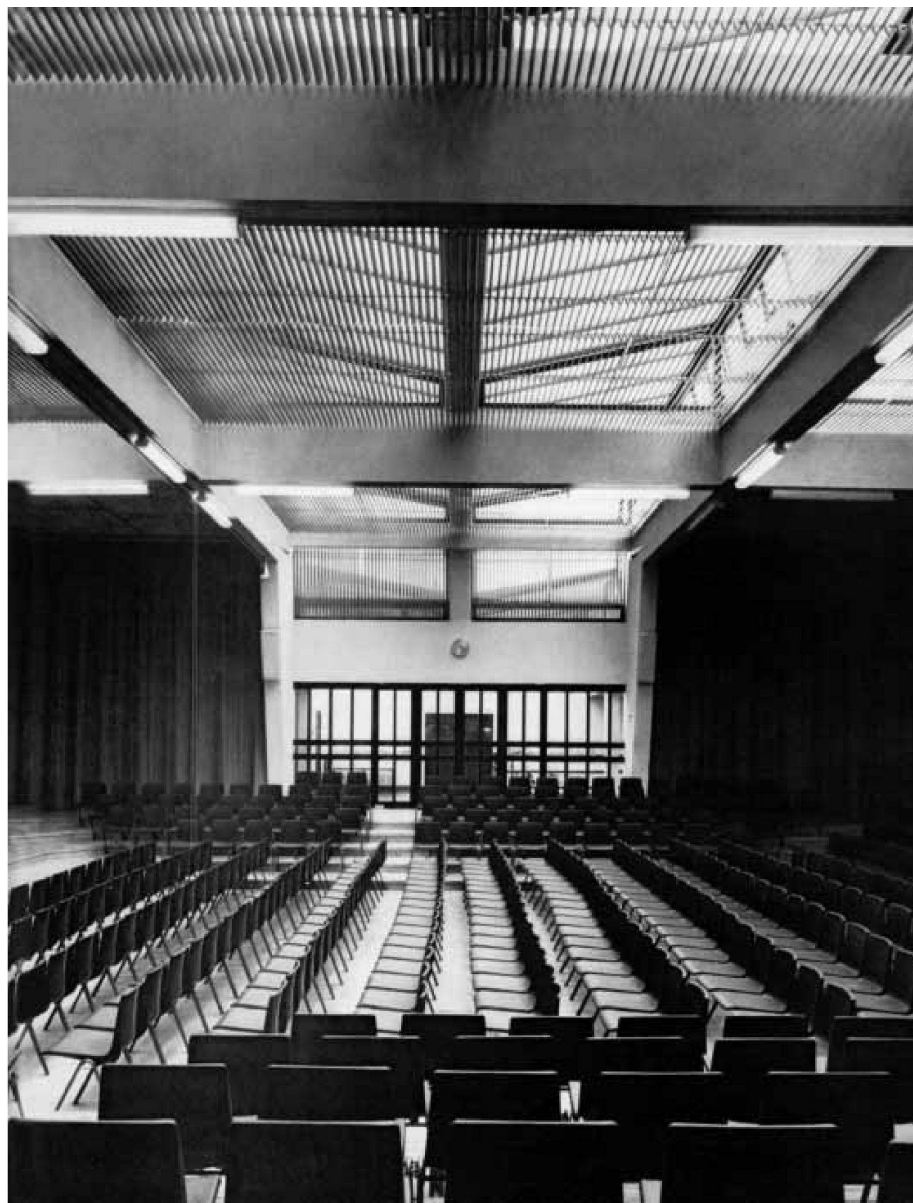
Aula. – Aus: The Architectural Review 150, 893 | 1971
