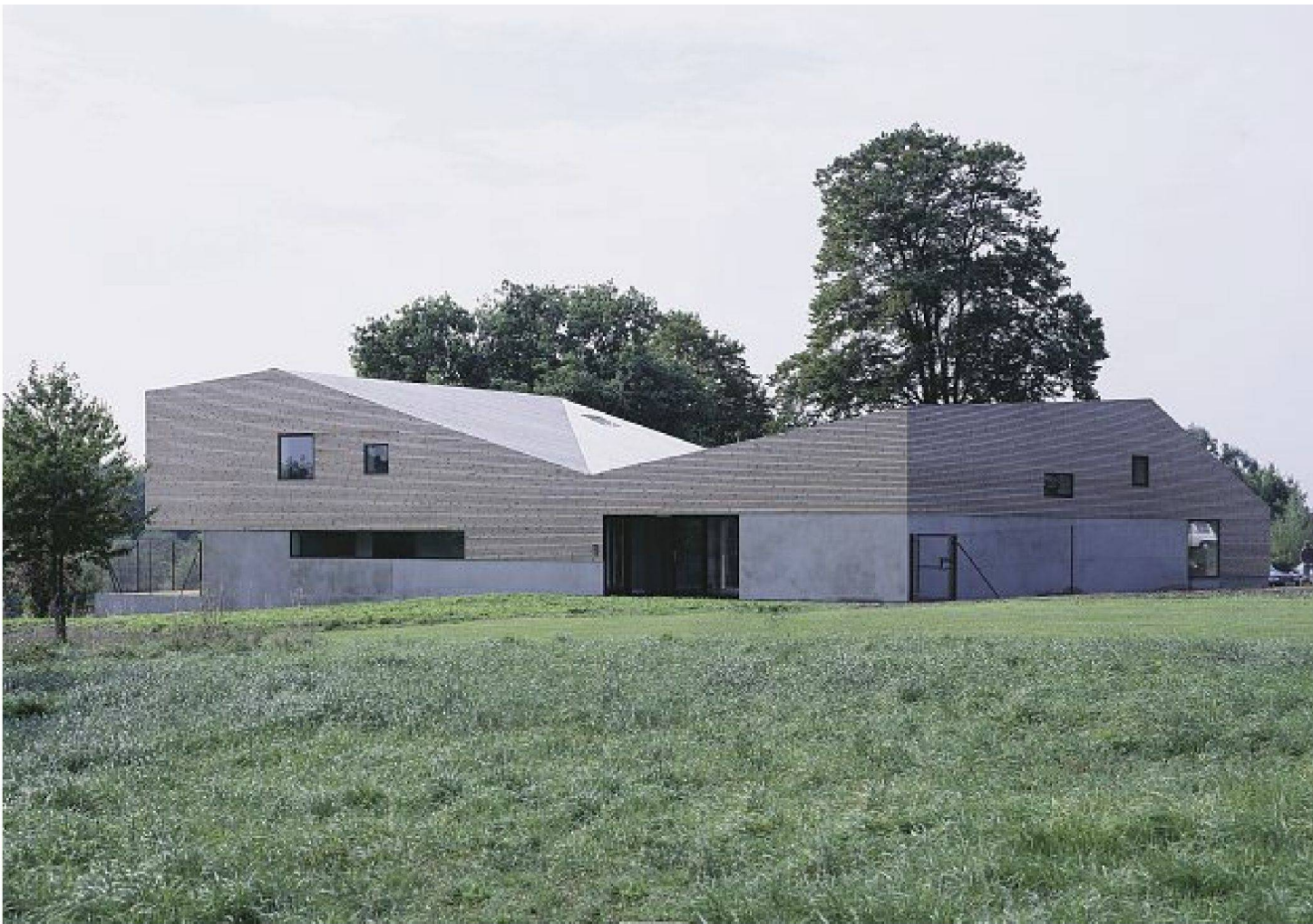
St Anne's Community & Sure Start Centre, Colchester, 2006. – Bild: Edmund Sumner
