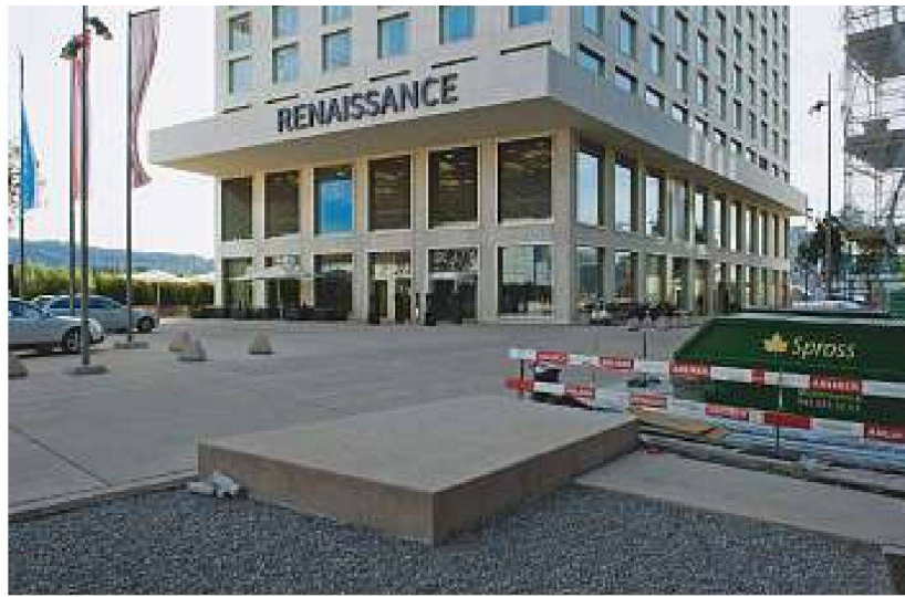
Mobimo Tower, Erdgeschoss
