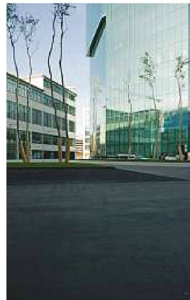
Sockel des Prime Tower
