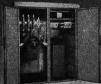
Transformatorstation in Freiluftkabine 50 kVA, 1000/220 V
