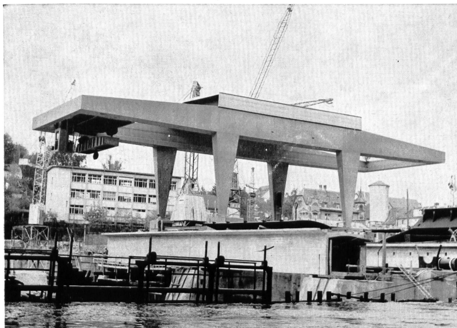
120 t Portalkran KW Schaffhausen
