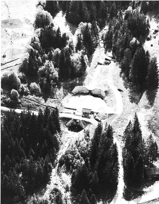
Figure 2. Erlentobel gauging station: measuring sill with nine built-in hydrophonic sensors to determine beginning and end of sediment transport, and to estimate thickness of sediment bearing layer.
