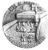
22 Stauwau Zervreila; 1954–1957 KW Zervreila AG, Vals; Valser Rhein; Zervreilasee
