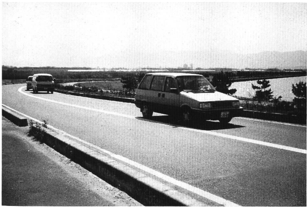
Figure 3. Embankment along the shore of Lake Biwa.
