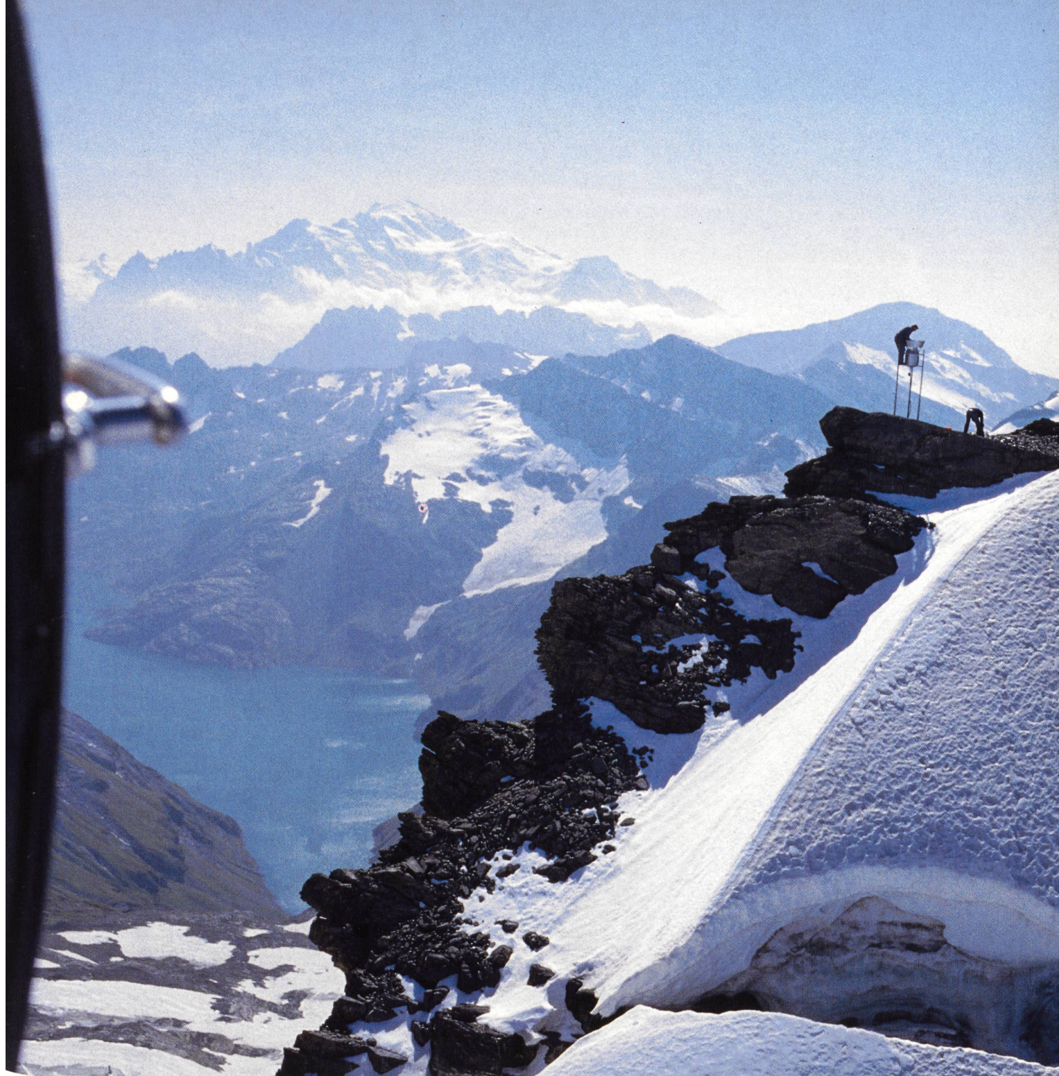
Installation of a pluviometer. Col de la Tour Sallière, 2891 m, in front of the Mont-Blanc, Switzerland.
