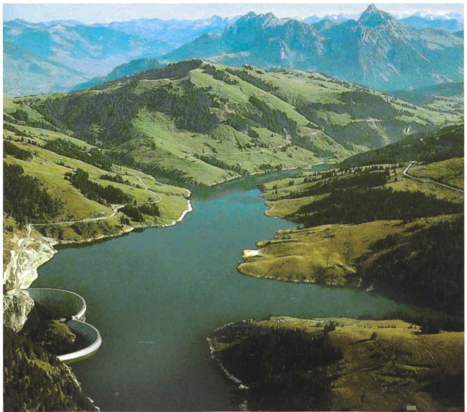
Figure 1. Hongrin dam and reservoir.
