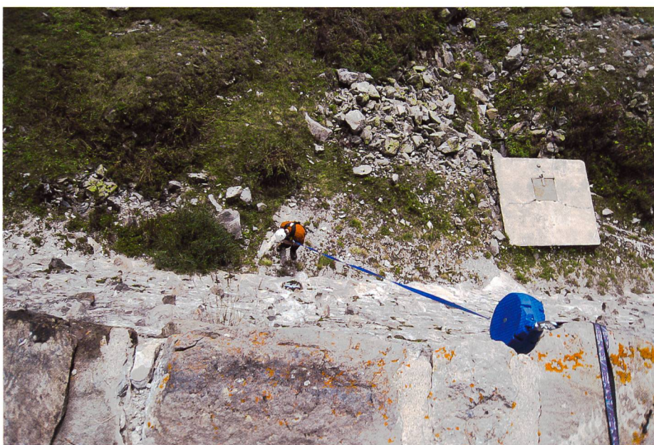
Figure 4. Controlling the dams surroundings.
