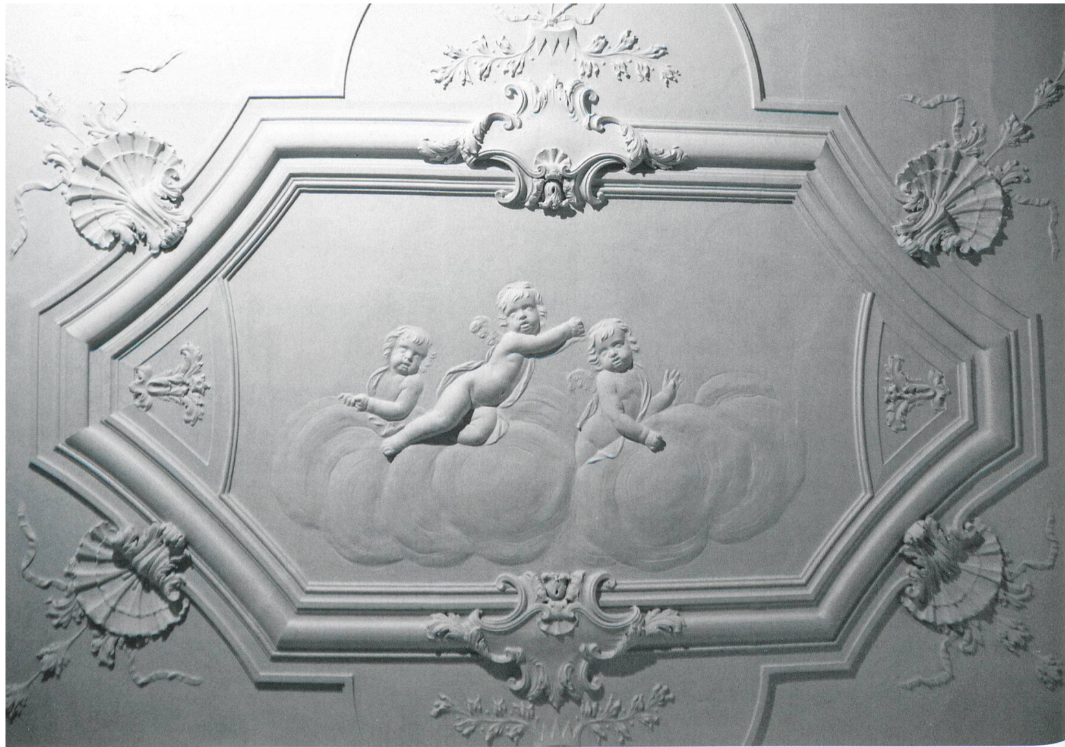
Fig. 11 Carlo Maria Pozzi, ceiling of the Retiradezimmer, Schloss Idstein, Hessen. Reproduced courtesy of the Pestalozzi Schule, Idstein.
